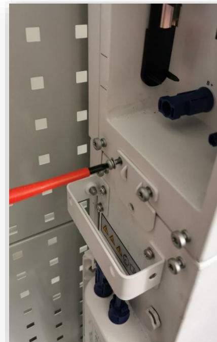
Fix power module to top battery left + right
