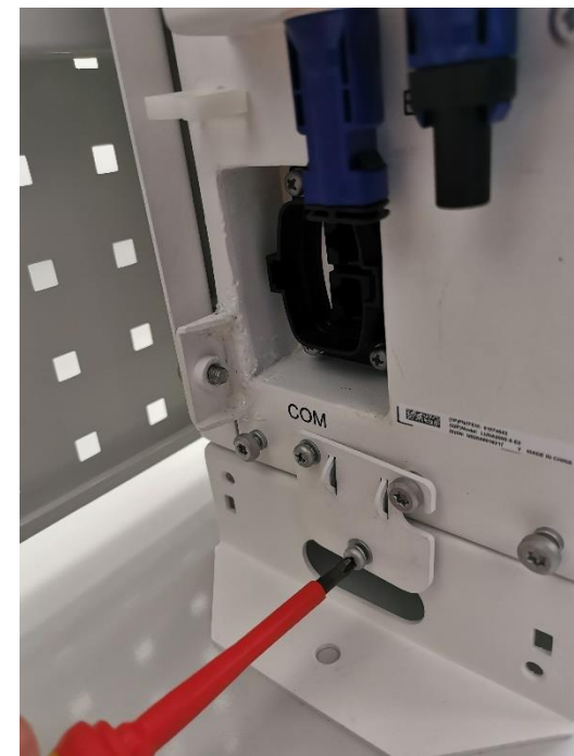
Fix battery to floor support left + right
